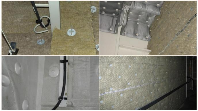
Easy and secure fastening of insulation wool through a combination of previously welded insulation pins / VBS pins and clips fitting exactly to the diameter of the welded insulation pins / VBS pins.
