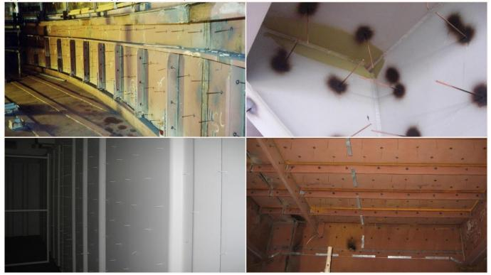
Easy and safe welding of insulation pins using drawn arc welding according to EN ISO 14555
